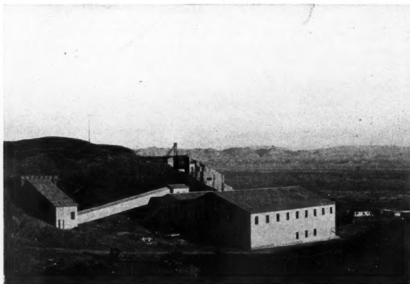
BLACK MAMMOTH Consolidated Mining Company's 100-ton cyanide mill at Silver Peak, Nev. The mine is about six miles away and the ore is transported to the mill in 10-ton trucks.
